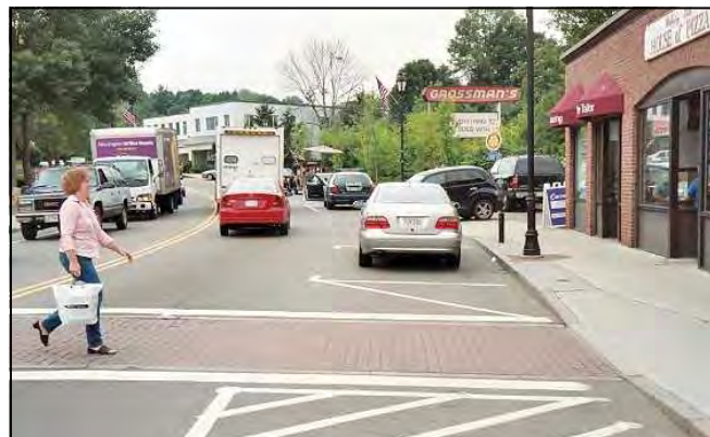
This photo represents a combination of both raised crosswalks and the addition of parallel on-street parking as traffic calming devices.
