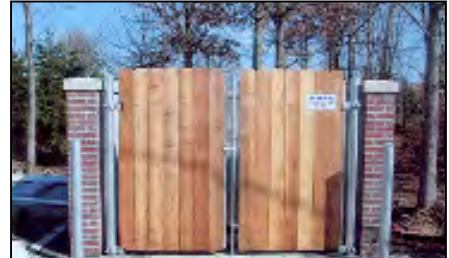
Dumpster screening featuring brick and wood elements.
