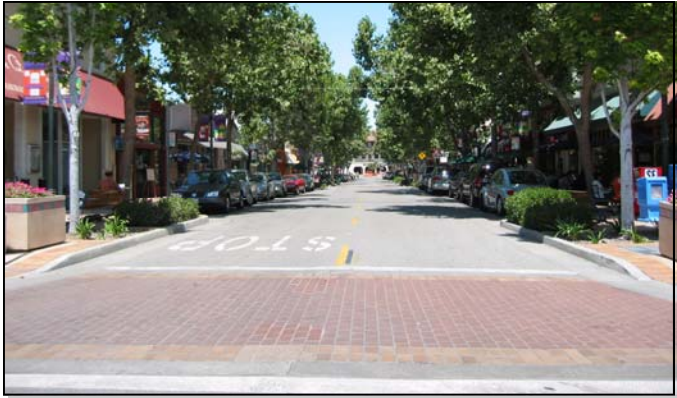
This photo illustrates the use of brick pavers to create a raised crosswalk. This provides for both traffic calming and adds an important streetscape element.
