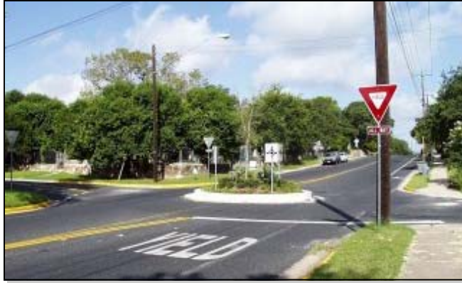
Shown above is a traffic circle. These designs provide for both traffic calming and present opportunities for landscaping and signage projects
