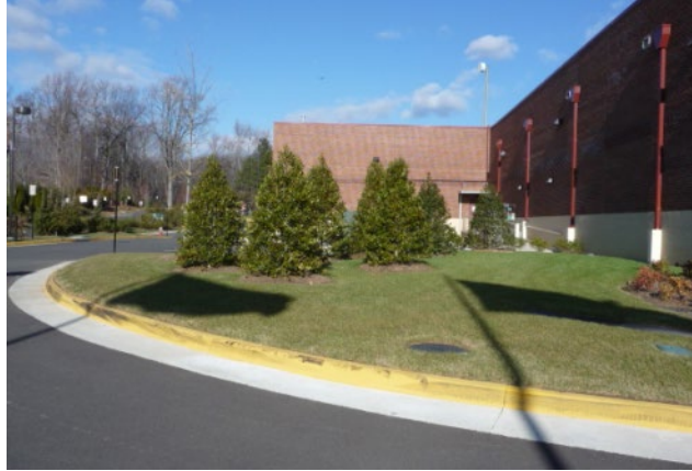
Figure 10-D: The above image illustrates a vegetative screen that hides HVAC equipment and a dumpster.
