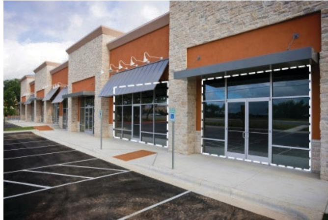
Figure 13-A: The window area is illustrated within the dashed line area for the two storefronts in the above image.
