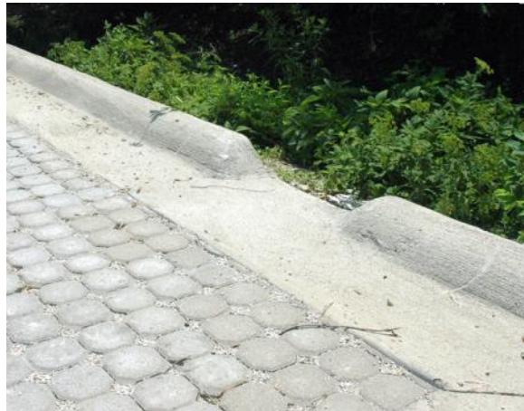
Figure 12-B: Cuts in the continuous curb allow for stormwater to be directed into landscaped areas.
