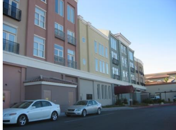
Figure 9-D: This figure shows two methods of using architectural features to create wall surface relief on wall elevations that are not the primary elevation.
