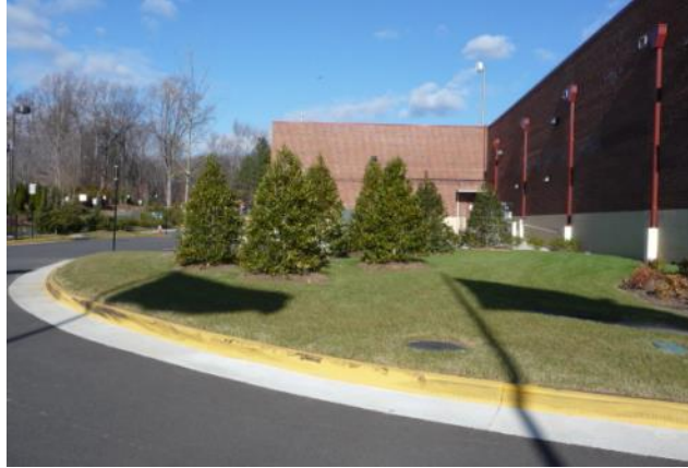
Figure 10-D: The above image illustrates a vegetative screen that hides HVAC equipment and a dumpster.
