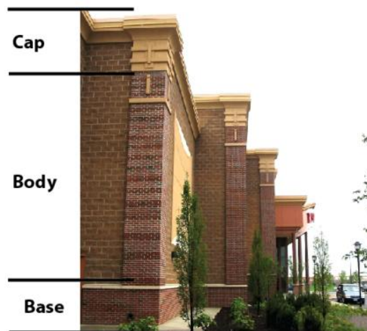
Figure 9-E: Image of a building with a clear, base, body, and cap
